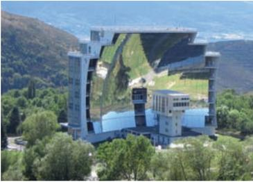
Labelled as "Great European Science Infrastructure", the Large Solar Furnace at Odeillo with a thermal power of 1000 kW, is one of the world's two largest solar furnaces. Put into operation in 1970, it can reach temperatures above 3,400 C°, without the input of polluting substances. The sunlight is
